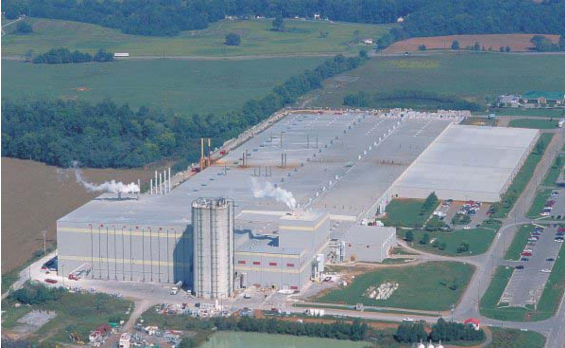
Figure 14. Photograph of a Large Ceramic Tile Manufacturing Facility.
